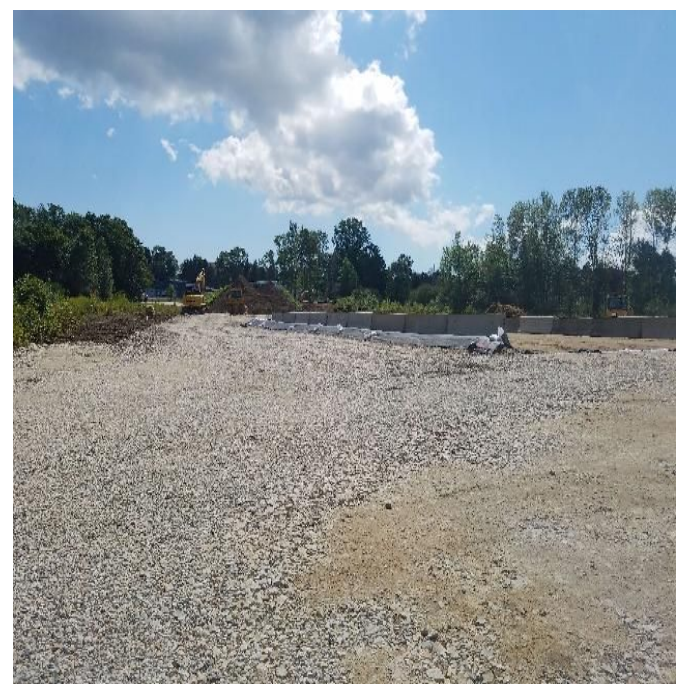
Fig 8: Shattuck Rd laydown yard, second basin. Viewing east. (9-3-19).
