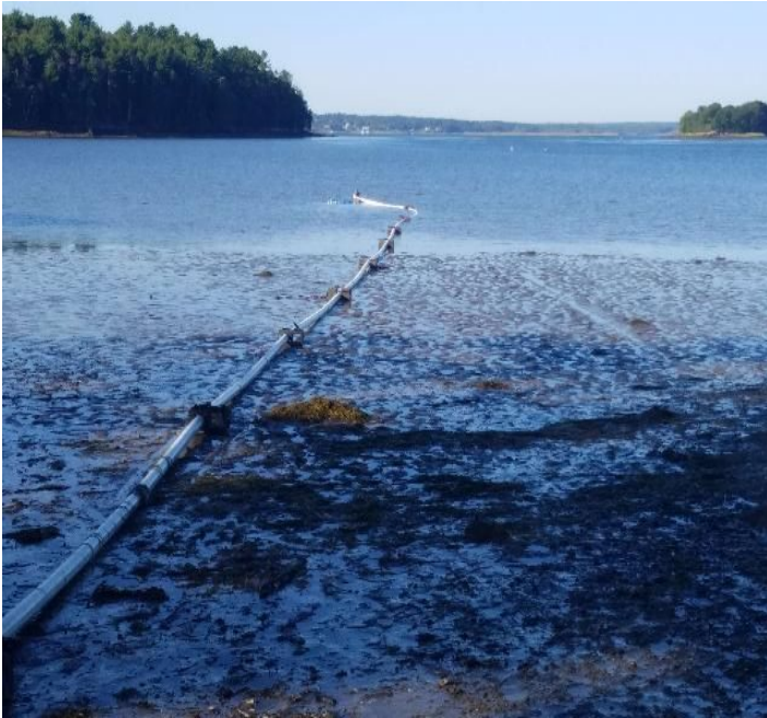
Fig 1: Boat ran over the PVC discharge pipe at Gundalow Landing. Viewing west. (8-30-19).
