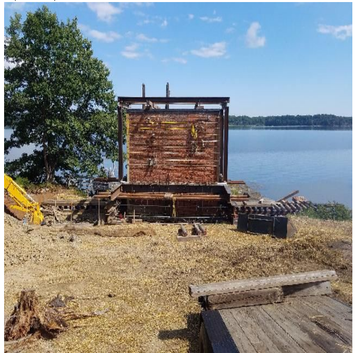
Fig 4 Cable house moved to temporary location. Viewing west. (9-3-19).
