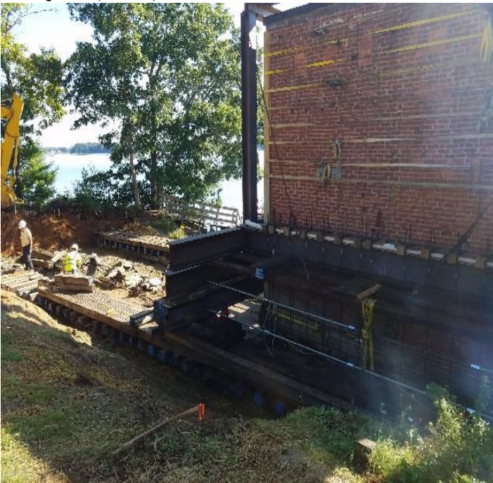
Fig 3: Gratan prepping to move the cable house. Viewing northwest. (9-3-19).
