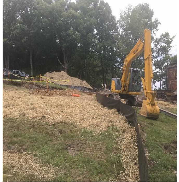
Fig 14: Silt fence installed downslope of Blu Rock excavation. Viewing south. (9-4-19).
