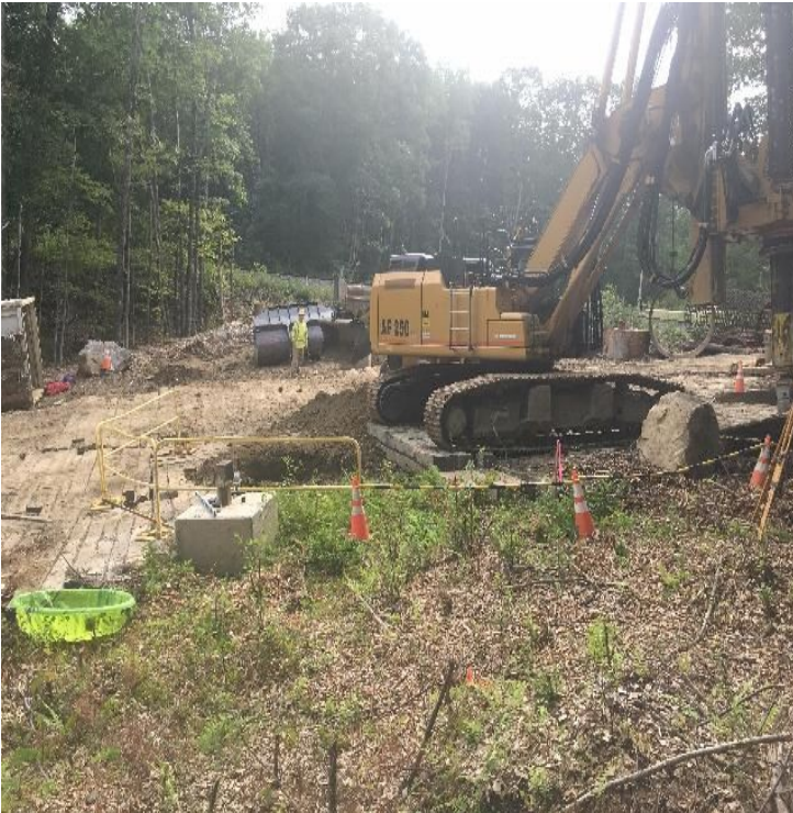
Fig 15: MJ drilling Str. 29. Viewing southeast. (9-4-19).
