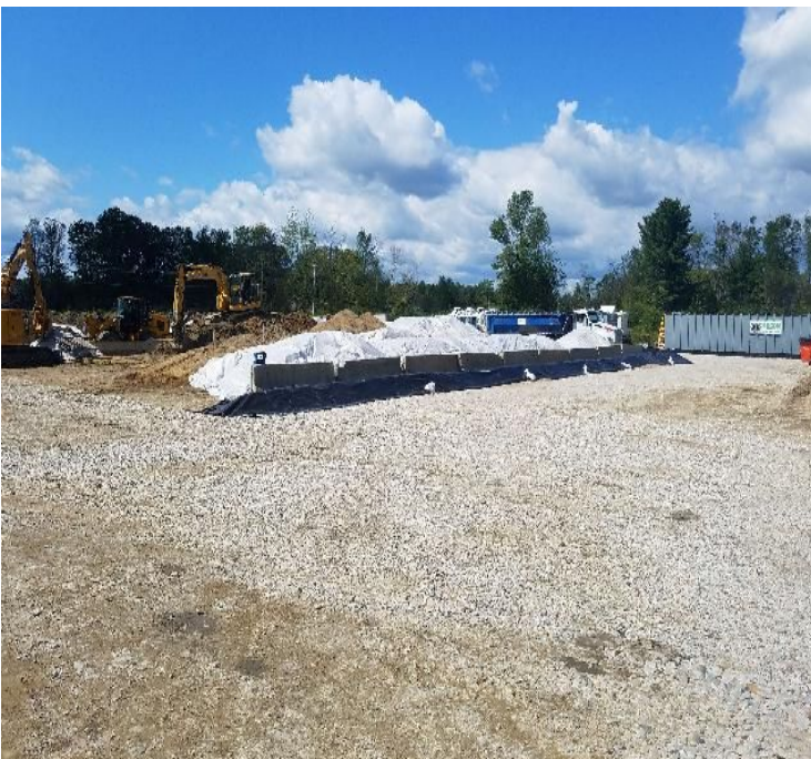
Fig 7: Shattuck Rd laydown yard, soil stockpiled in first bay. Viewing southwest. (9-3-19).
