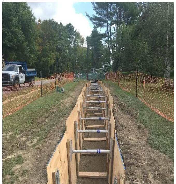
Fig 12: Underground cable trench along Gundalow Landing. Viewing east. (9-4-19).
