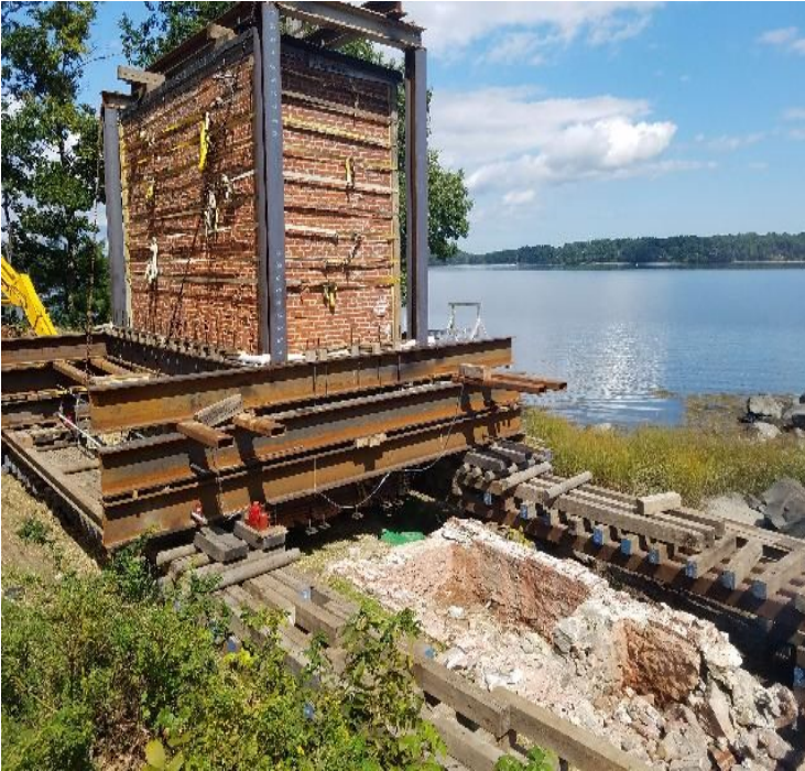
Fig 5: Cable house moved to temporary location. Viewing northwest. (9-3-19).
