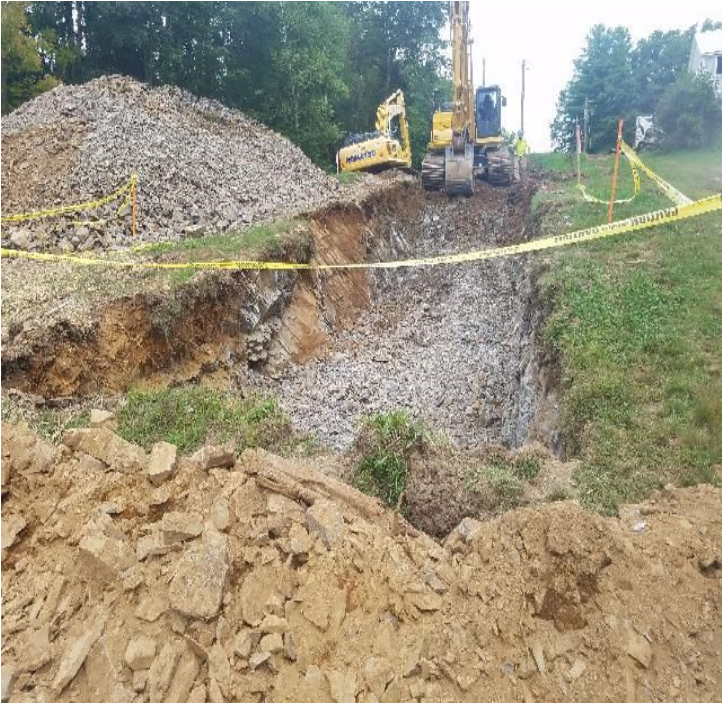
Fig 13: Blu Rock trenching at west side of Little Bay. Viewing east. (9-4-19).
