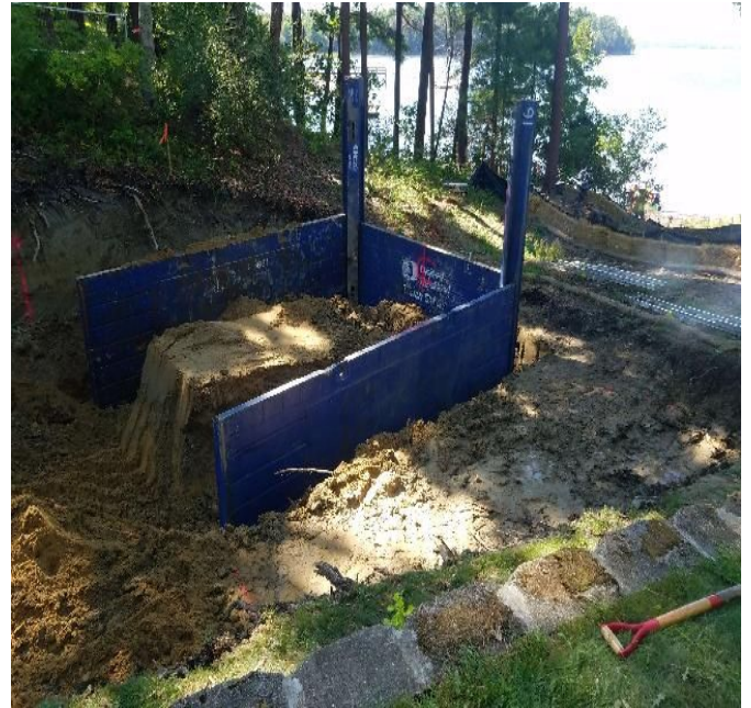
Fig 2: Trench box for manhole excavation. Viewing southwest. (8-30-19).
