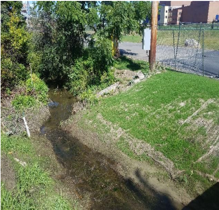
Fig 9: Upstream at College Brook. Viewing west. (8-24-19).
