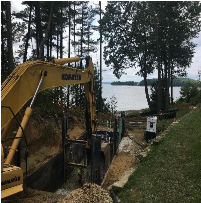
Fig 11: Manhole excavation at Gundalow. Viewing southwest. (9-4-19). east.
